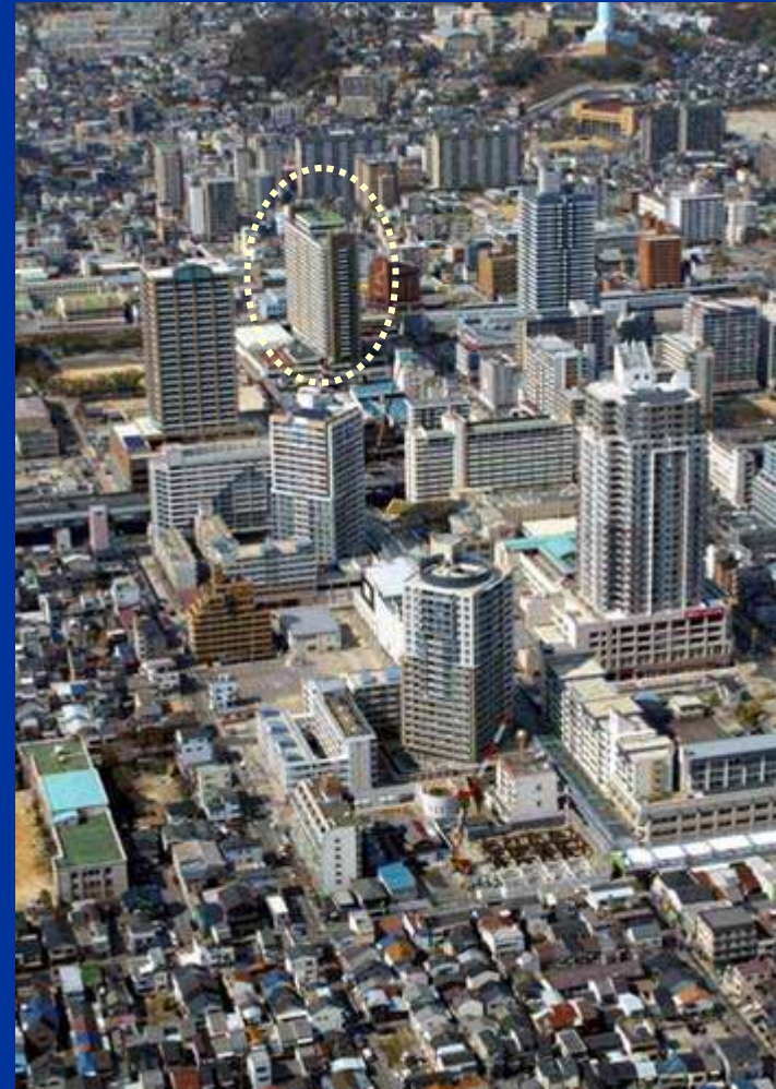
Overview of Shin-Nagata area after the implementation of the urban recovery projects (2005)
