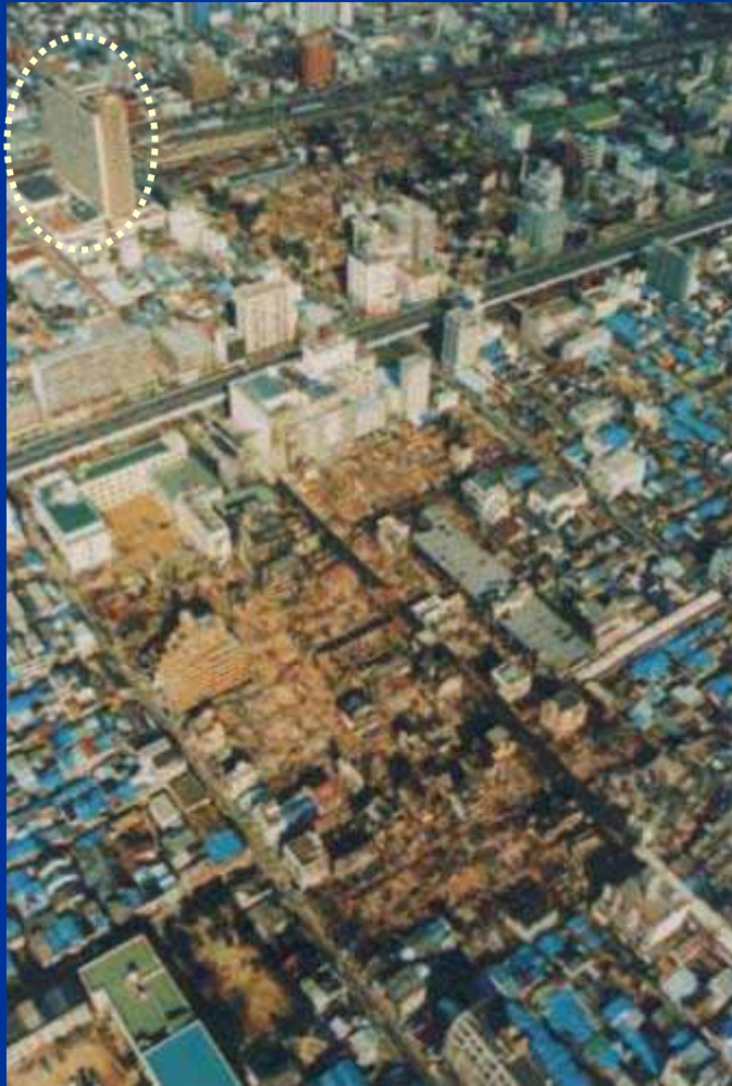
Overview of Shin-Nagata area immediately after the earthquake (January 1995)
